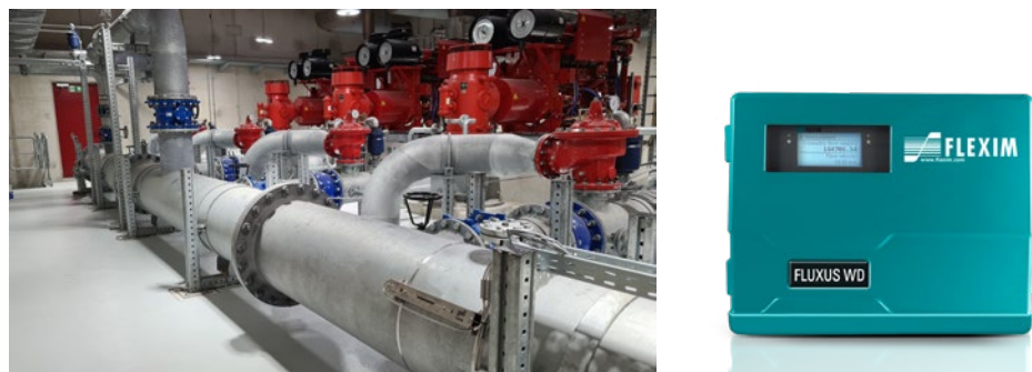
FIGURE 9.1 Flexim FLUXUS® 721 clamp-on ultrasonic flow meters can be used on a permanent or temporary basis to analyze water flow.
